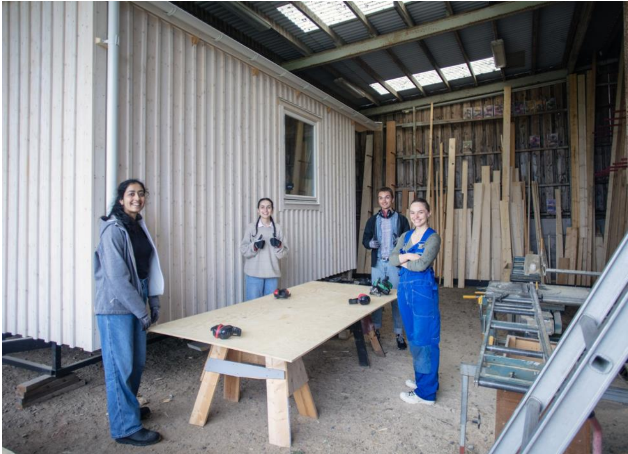
Students doing construction work at Egnahem Fabriken. Photograph Carrie Bobo
